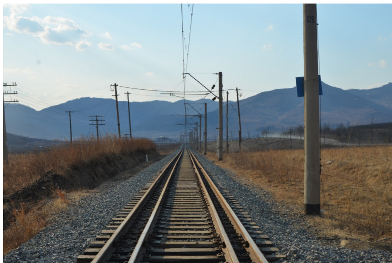
The double-gauge railway connecting Russia and North Korea.
