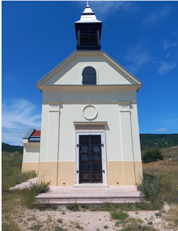
A restored 19th century German chapel outside of Budapest. (Philip Wasielewski)
