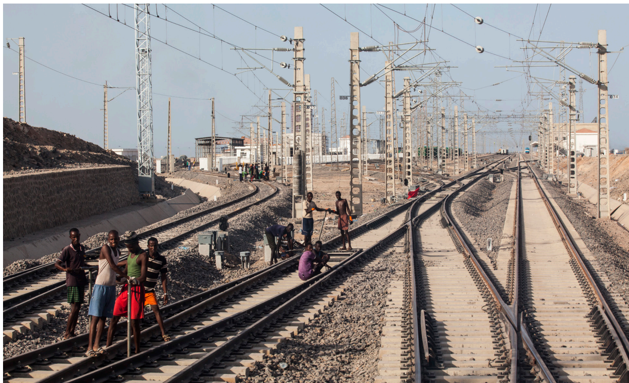
Local constructors maintain the Addis Ababa-Djibouti railway at the railway station of Djibouti city, Djibouti, 29 December 2016. After four years' construction, the Addis Ababa-Djibouti railway, the longest electric railway in Africa, crossing Ethiopia and Djibouti, was officially opened on October 5, 2016. Africa's first cross-border electric railway was built by Chinese enterprises and the opening of the railway marks a significant milestone in the development of the two countries. (REUTERS)
